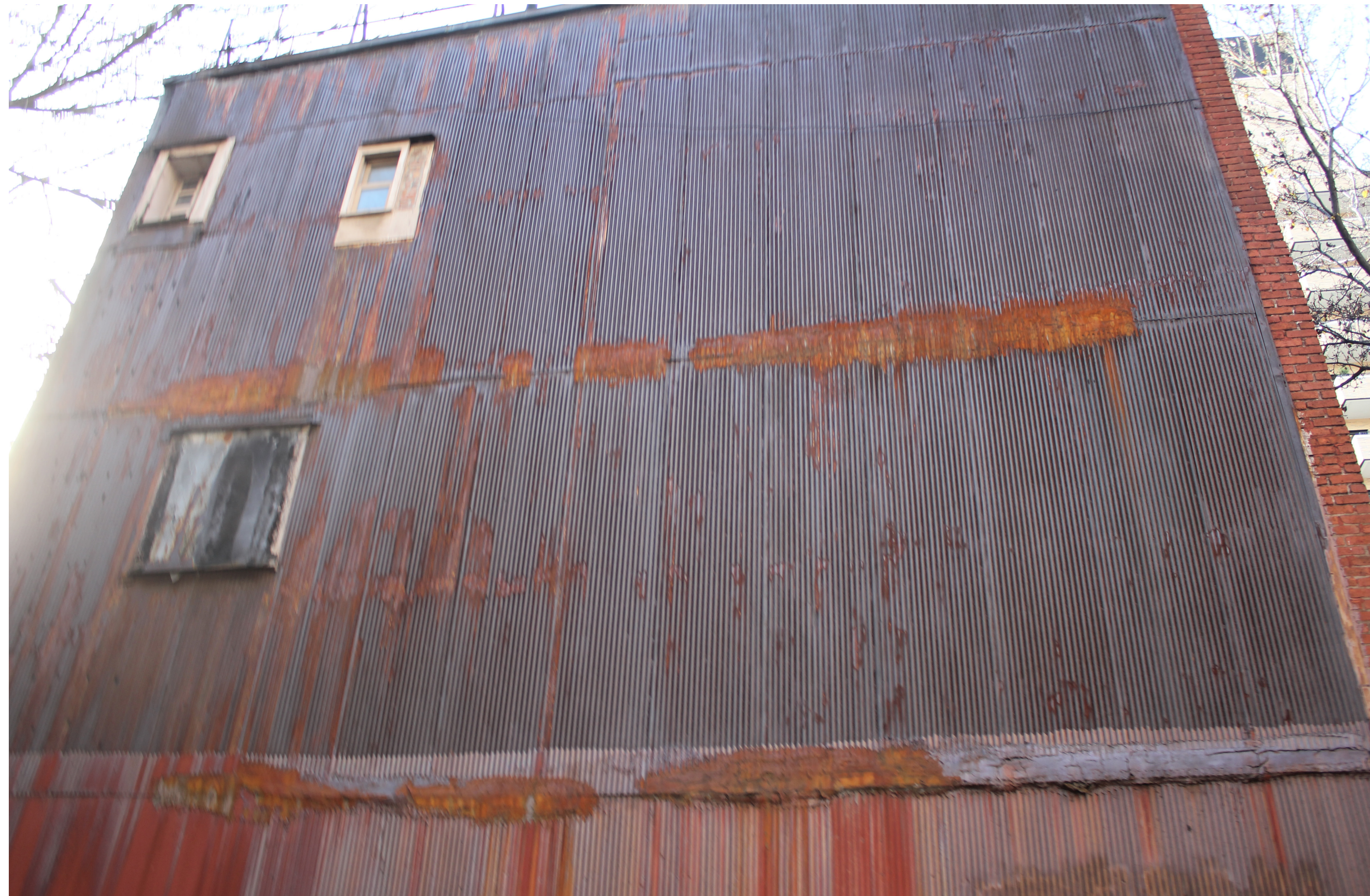
metal panel, view from neighboring lot
