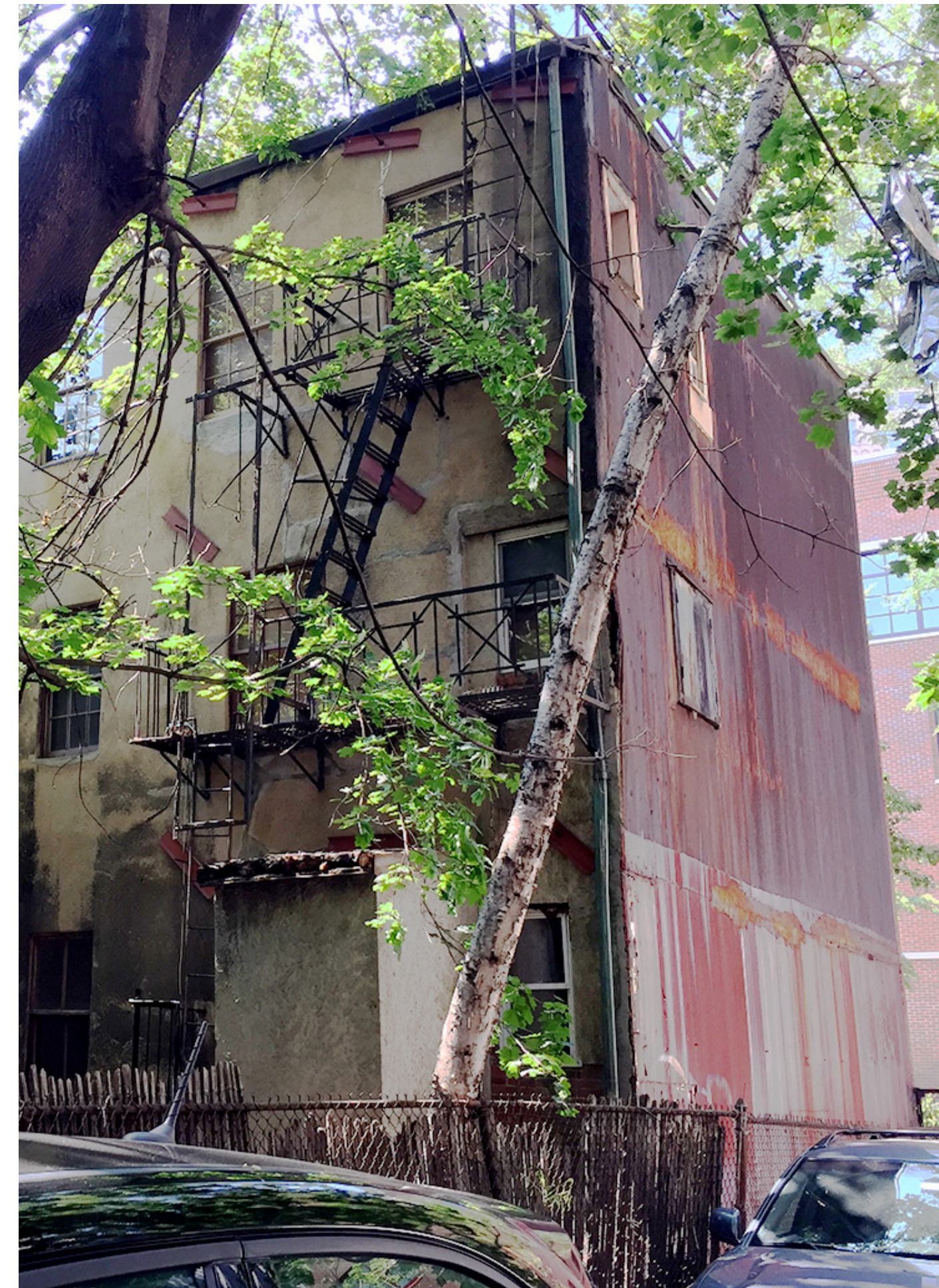
metal panel, view from rear
