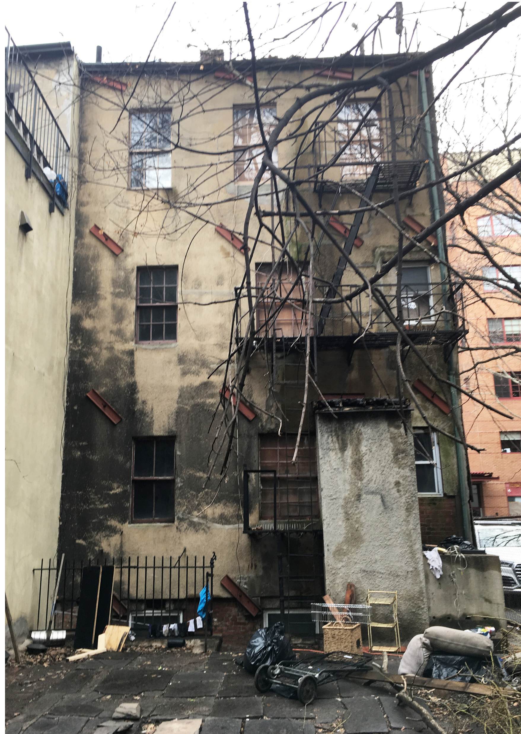
Rear view of 85 Sullivan Street
