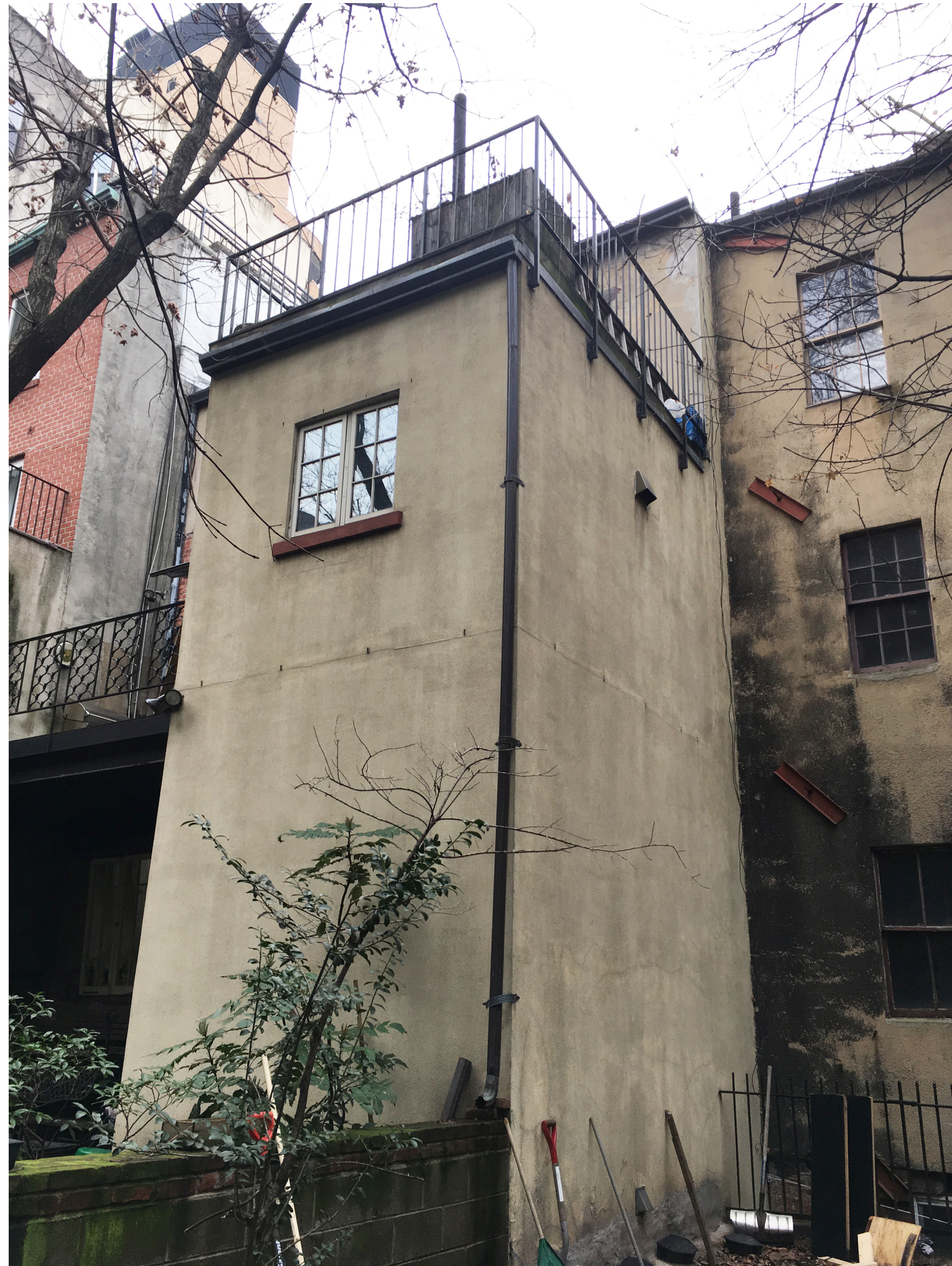
Two-story extension at 83 Sullivan Street
