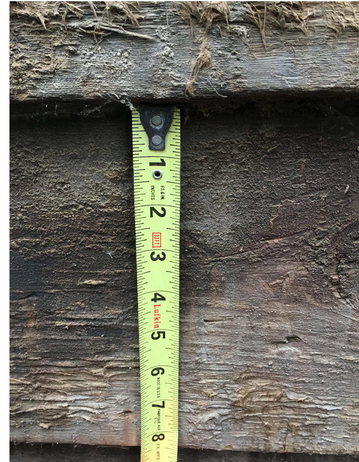
typical height of clapboard siding
