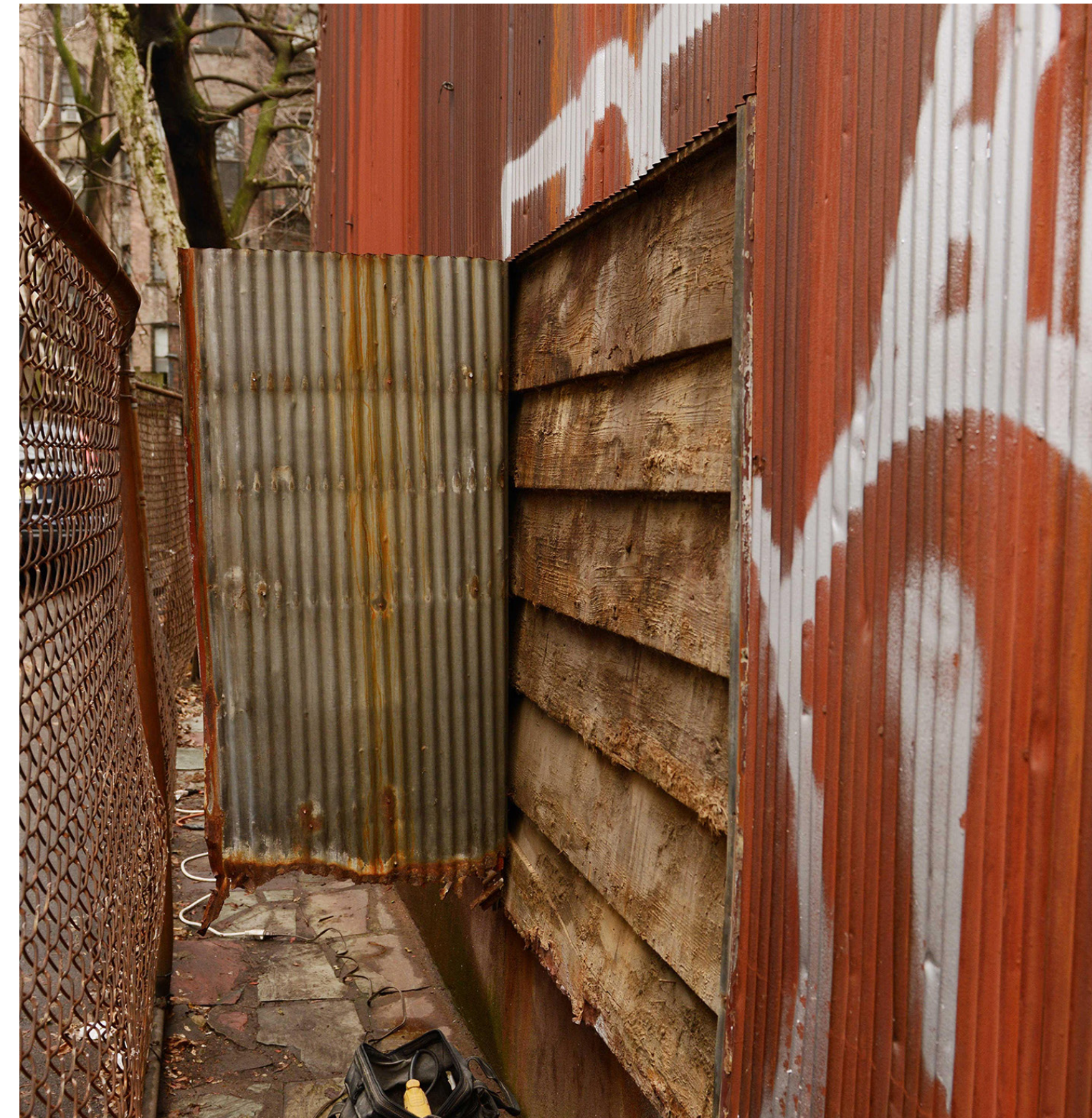
view of clapboard siding under metal panel
