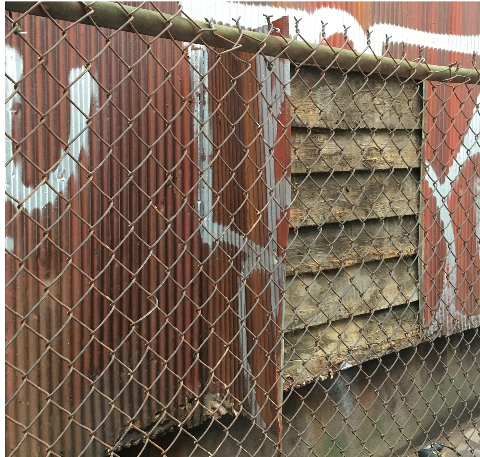
view of clapboard siding under metal panel
