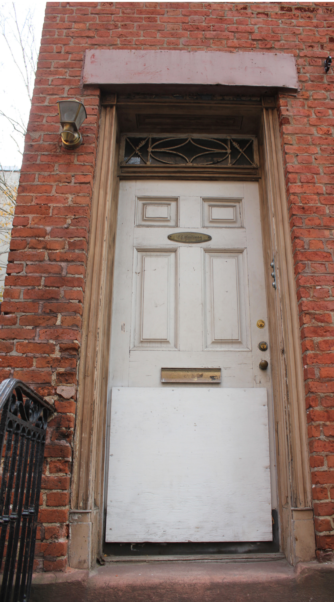
Existing entry door
